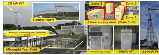
100 kW Autonomous Micro-grid Demonstration System
